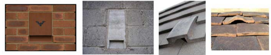
examples of bat tiles, bricks, integrated bat boxes from BCT http://www.bats.org.uk/pages/bat_boxes.html
